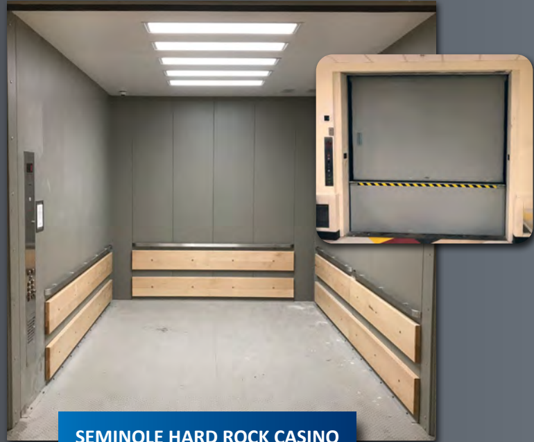
SEMINOLE HARD ROCK CASINO Ft. Lauderdale, FL Twin Jack Holeless 10,000 lb. Capacity
