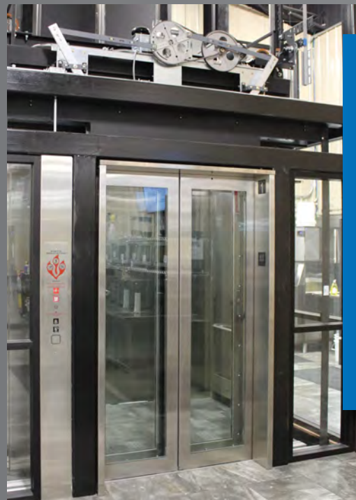
MEI Headquarters - Mankato, MN - Glass panels set in SS #4 framing, concealed vents, 1 1/2" round handrail with returned ends, SS #4 fronts and a SS #4 drop ceiling with low voltage LED lights
