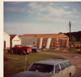
This structure is currently part of the main entry, front office.
